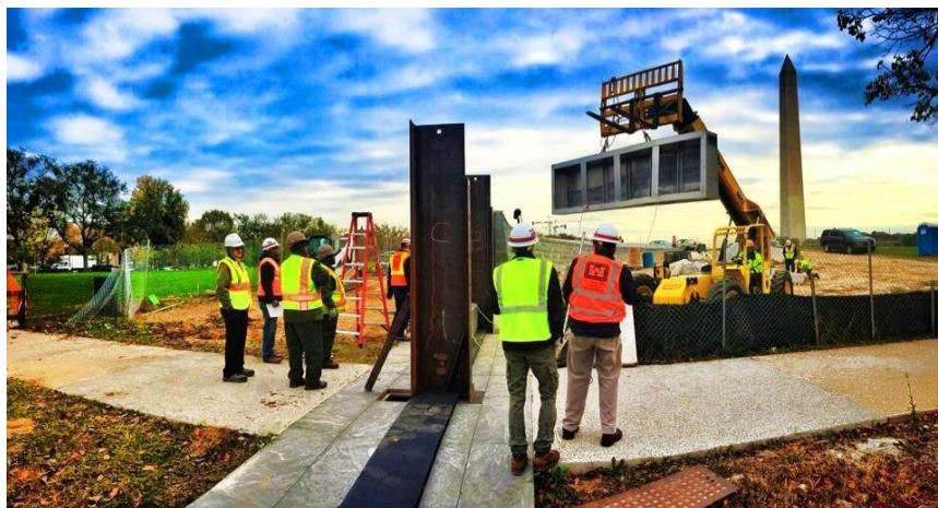
Installation of the newly constructed 17 th St Closure October 31, 2014 – photo USACE
