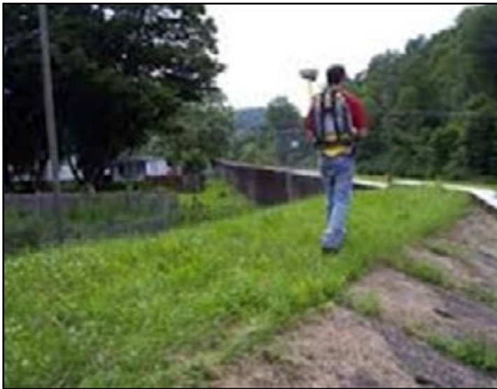
Inspector walking the levee's crest
