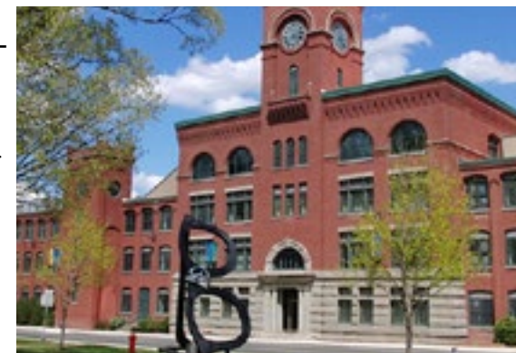
Executive Management Training Center in Southbridge, MA
