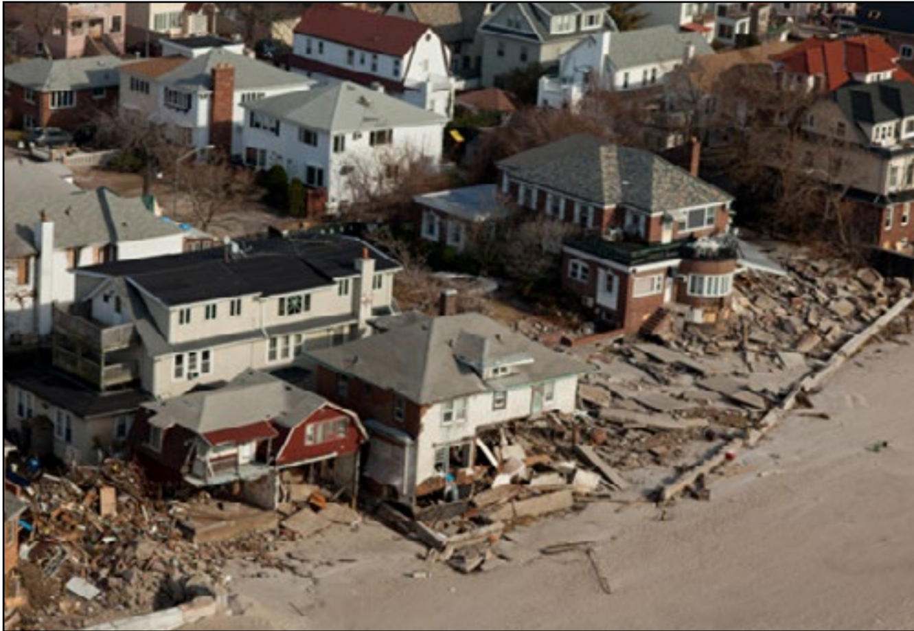
Coney Island home moved off its foundation by Hurricane Sandy. The waves and surge damaged thousands of homes on east coast. Photo from FEMA/Andrea Booher
